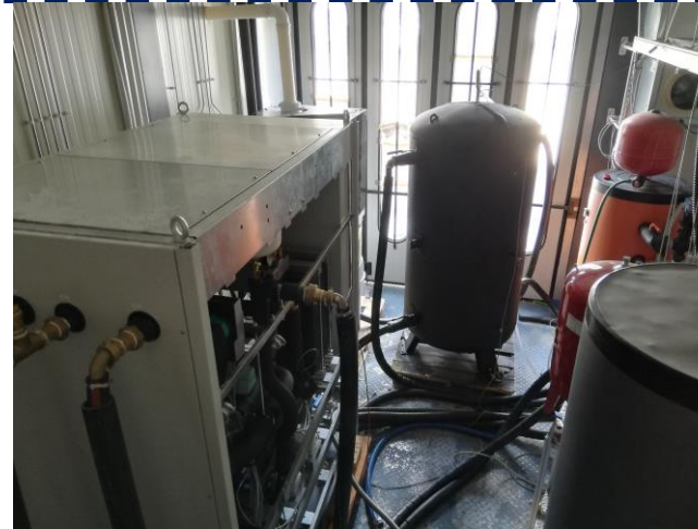
Geothermal Gas-driven heat pump (up to 10 kW heat)
