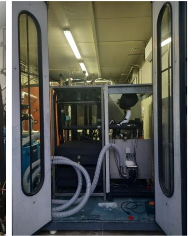
Parallel commercial sorption/propan compression (up to 40 kW cool)
