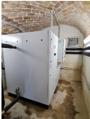
Geothermal gas-driven adsorption HP installation in a demo in Italy
