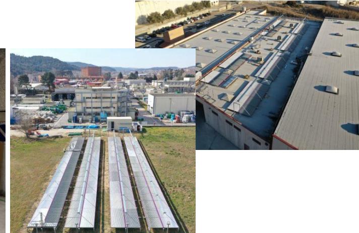
Hybrid heat pump integration in a civic centre in Spain driven by solar thermal collectors
