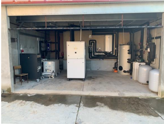
Geothermal gas-driven adsorption HP installation in a demo in Italy
