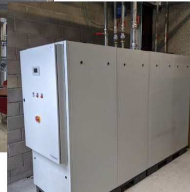
Hybrid heat pump integration in a civic centre in Spain driven by solar thermal collectors
