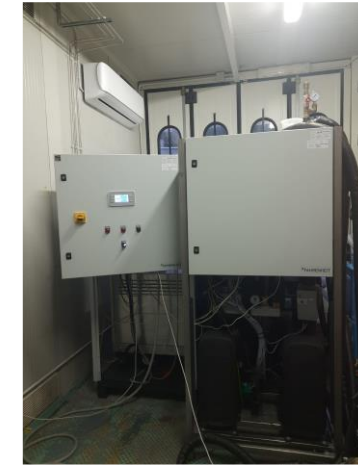
Parallel commercial sorption/propan compression (up to 40 kW cool)
