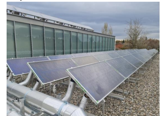
Hybrid heat pump integration in a civic centre in Spain driven by solar thermal collectors
